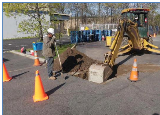
PHOTO: Teterboro, NJ: Clean-up of hazardous waste begins, decades after property seller's sworn statement that hazardous waste operations did not take place at site during his ownership.
